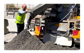
Unload the granulated materials after the treatment in a covered area in layers, no more than 25 cm thick;
