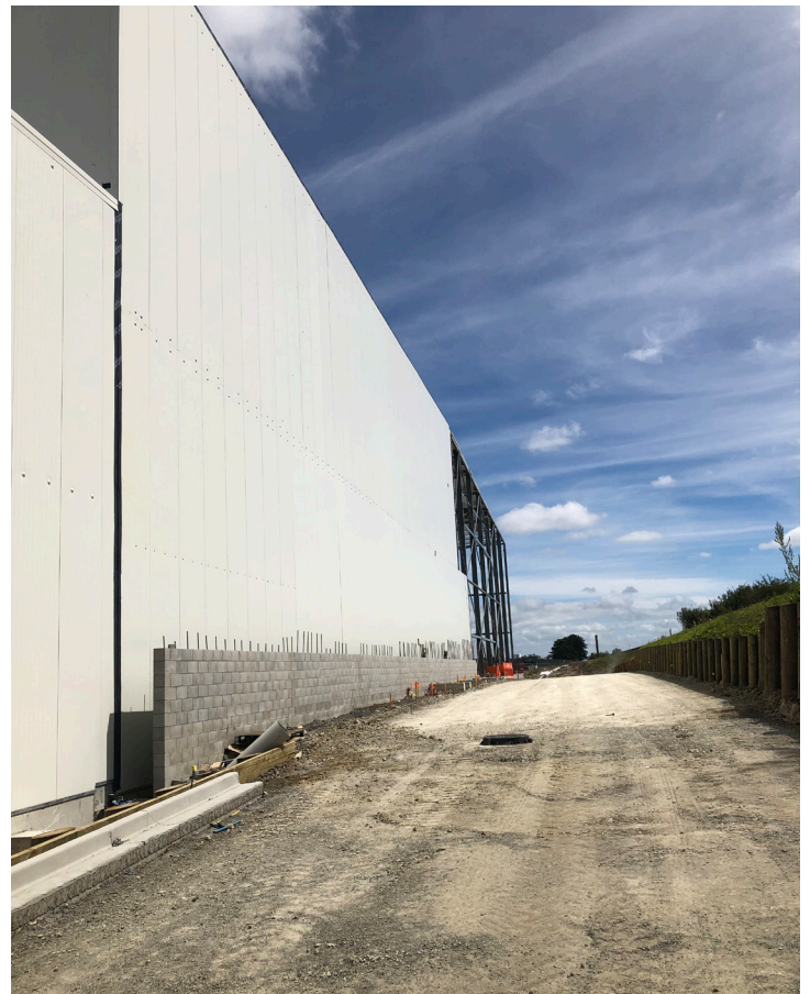
10,000m 2 Roofing - Kingspan Insulation panel
