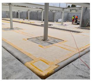
SikaProof® A-12 installed prior to floor concrete pour
