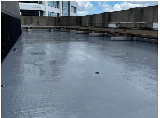
Completed. A seamless, waterproof membrane.
