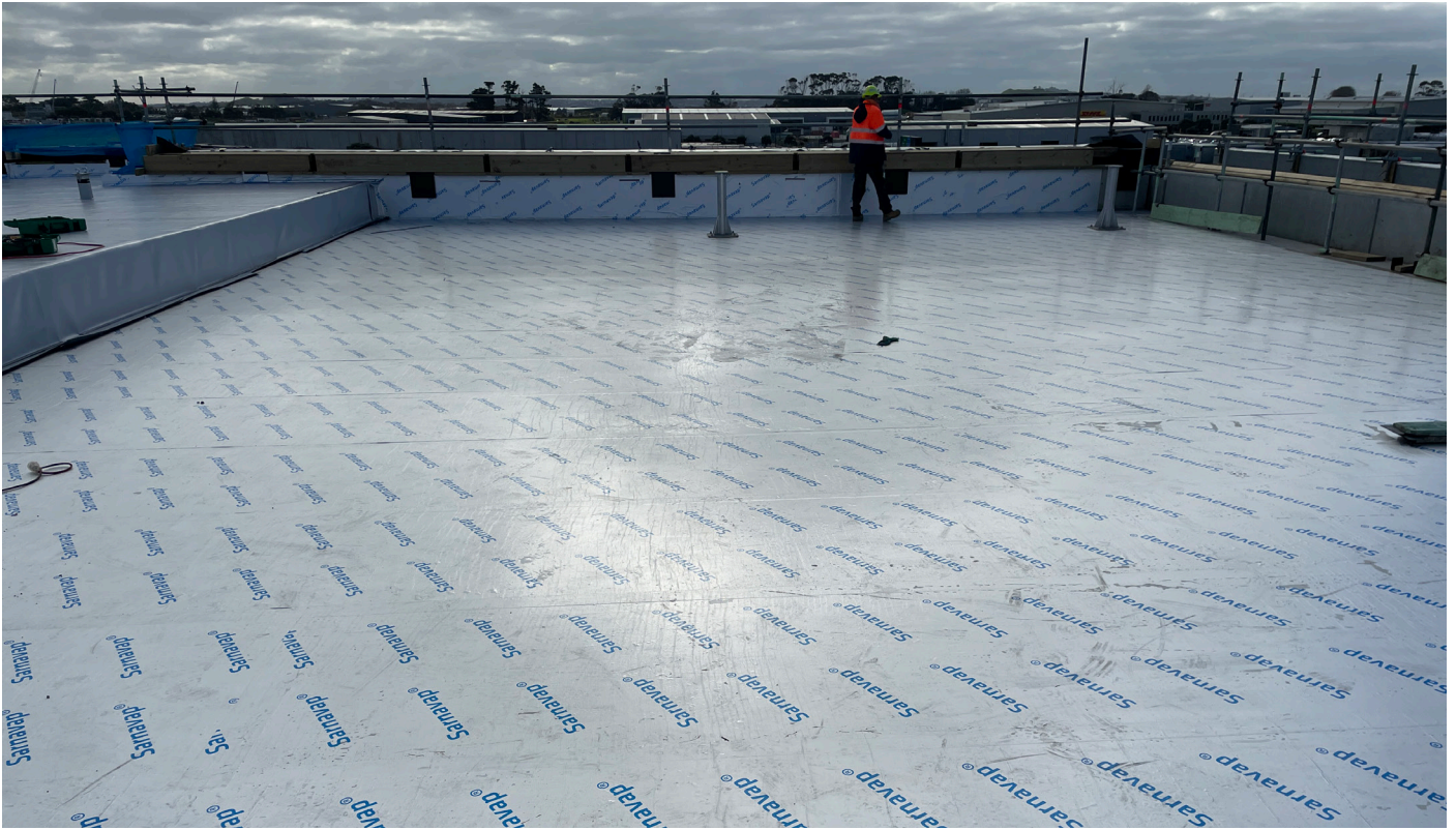
Sarnavap-5800 SA vapour barrier applied to the flat concrete substrate.
