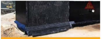
Minimum 100mm diameter drainage coil Minimum fall of 1 to 200
