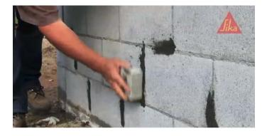
Once the holes have been filled, give it time to dry, then use your rubbing stone to smooth off the repaired areas
