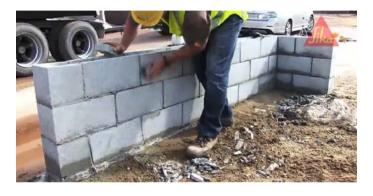
Then smooth the blocks down with either a rubbing stone, or a piece of concrete block will do
