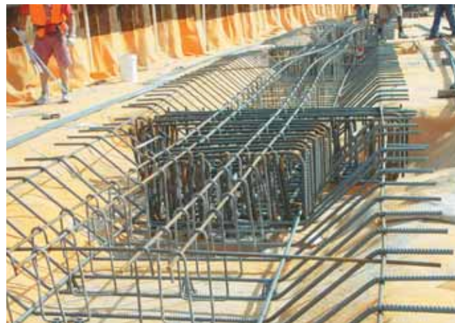
SikaProof Bentonite Basement Waterproofing Application
