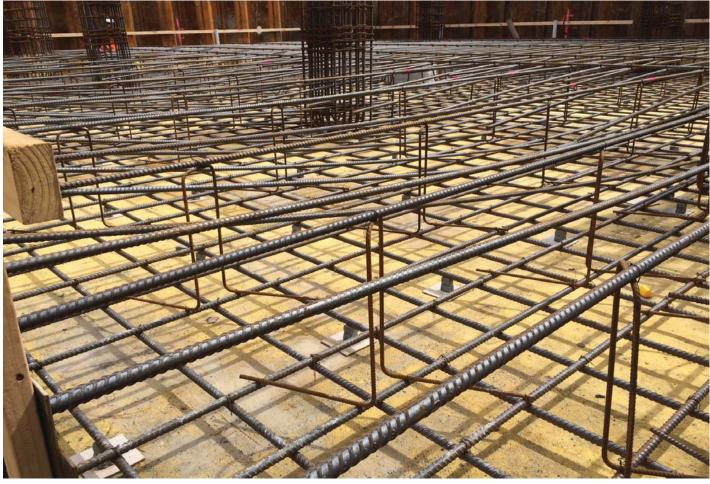
Amount of reinforcement being placed does not damage the waterproofing membrane
