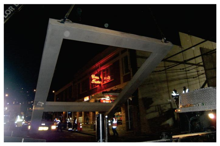
Because of the early strength achieved with Sika ViscoCrete-2100, the evening lifting and transportation of the panels was executed without damage to the panels or any delays to the programmed road closure
