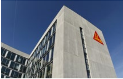
Fig. 8.12.2: With a wide variety of formwork and treatments available, almost any concrete finish can be created, included mirror smooth, plain timber board or other patterns, for example bush hammered or exposed aggregate etc..
