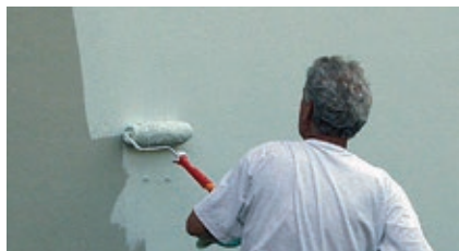
Fig. 8.8.2: As resistance of concrete against chemical attack is limited, protective coatings are often used for external protection. Epoxy resin-based protective coatings are applied over the entire surface following reprofiling of the concrete surface with sulfate-resistant repair mortar enhanced with synthetic material.
