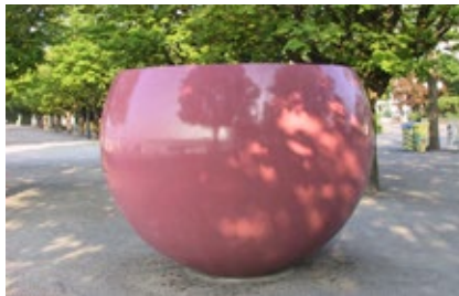
Fig. 8.12.1: Due to the development of SCC (self-compacting concrete), design and construction potential is now almost unlimited, and with special formwork technology and/or specific concrete admixtures, high quality finishes can be achieved even in the most difficult areas.
