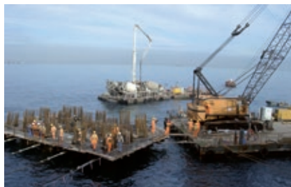
Fig. 8.14.1: When using underwater concrete, the placing and working conditions are very often complex, which is why these concretes often also need an extended working time.
