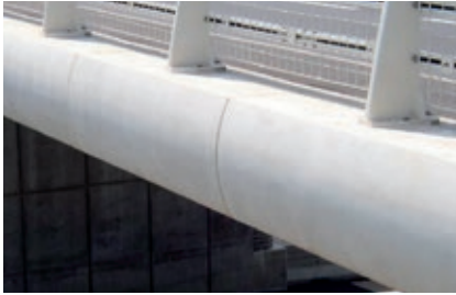
Fig. 8.9.4: Highly stressed building components such as columns and beams are made of high strength concrete. High resistance to external influences also makes high strength concrete an ideal protective coating for exposed construction elements.
