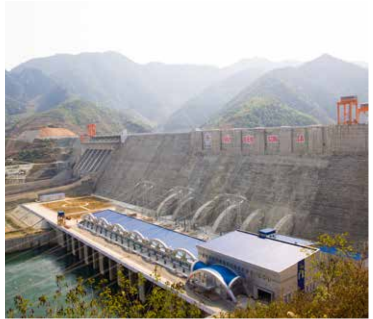
SON LA HYDROPOWER PROJECT, VIETNAM
