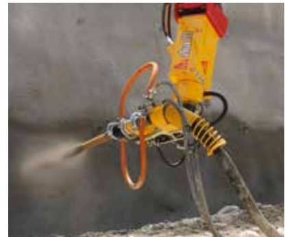
2. Slopes Stabilization, Page 12
