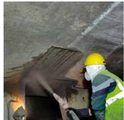
CONCRETE PROTECTION AND REFURBISHMENT
