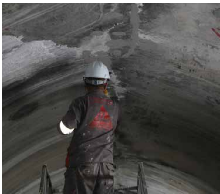
MOSUL DAM, IRAQ
