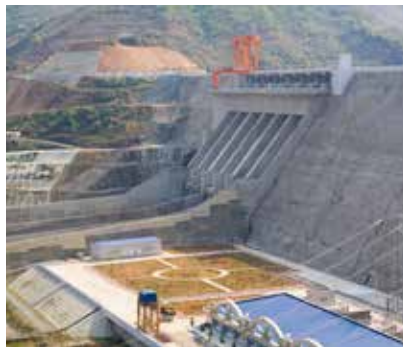
3. Spillway & Intake Structures, Page 13
