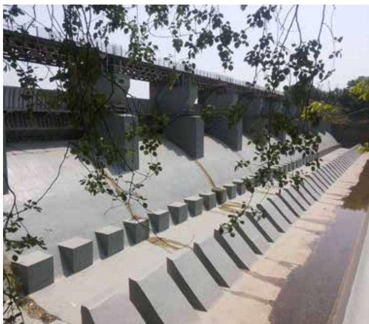
MANDIRA DAM, INDIA
