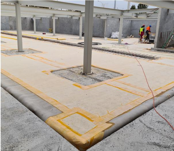
*SikaProof® A-12 installed prior to floor concrete pour*
