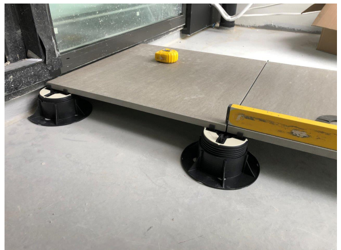
Placing tiles over Sikafloor®400 N Elastic, cured
