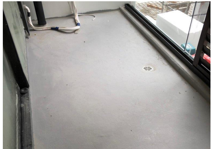
Sikafloor®-400 N Elastic installed on 90 Balconies
