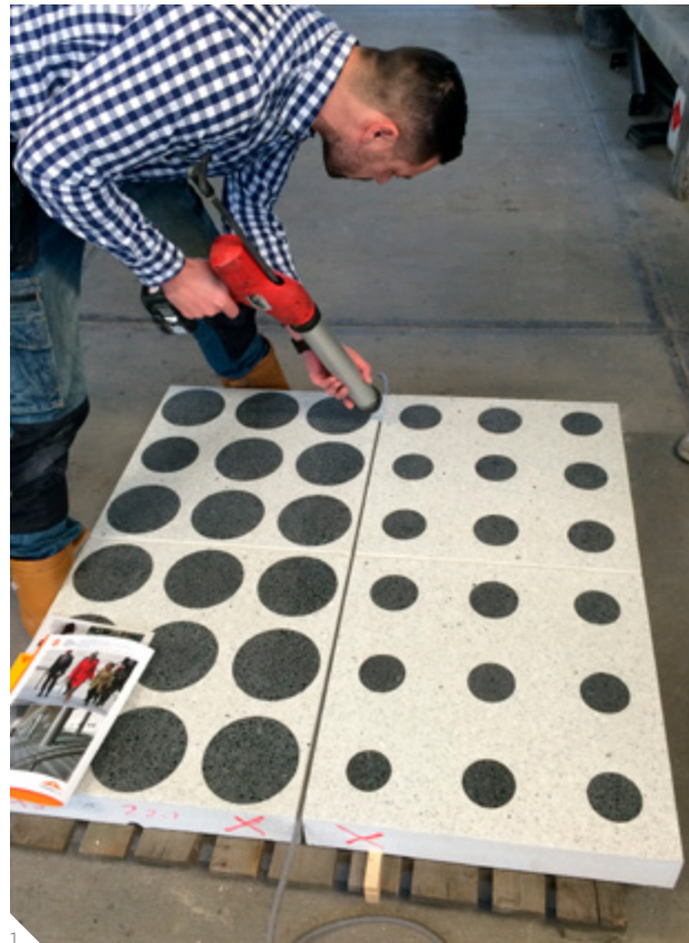
1 After installing the baker rod and applying with Sika® Primer-3N for optimal adhesion, the joint is sealed by Sikasil®-Pool. 2 The separate Terazzo concrete pieces before installing.
