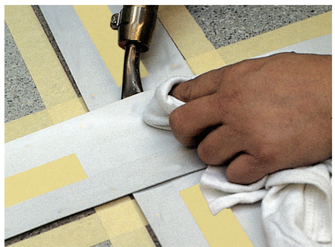
Hot air welding of joint details
