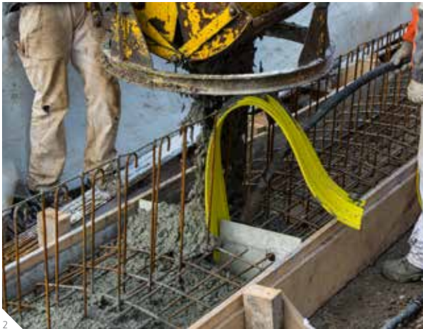
2 Sika White Box concept/Watertight concrete
