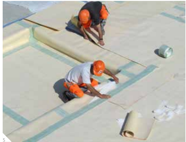
5 Fully bonded sheet membranes
