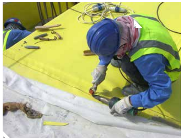
6 Compartmentalized sheet membrane systems
