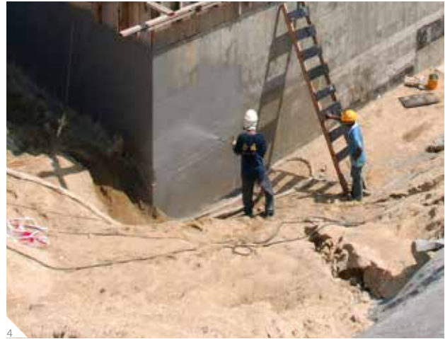
4 Liquid applied reactive membranes (PUR/PUA)
