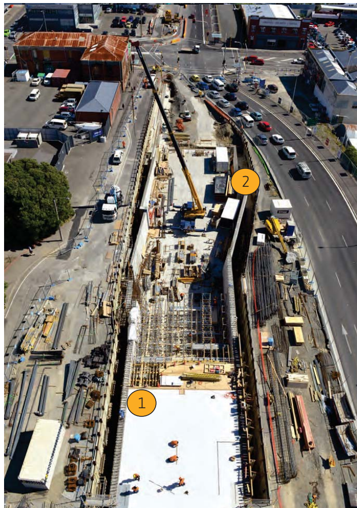
1. Tunnel roof taking shape 2. Sika Control 40 was used to cast the walls
