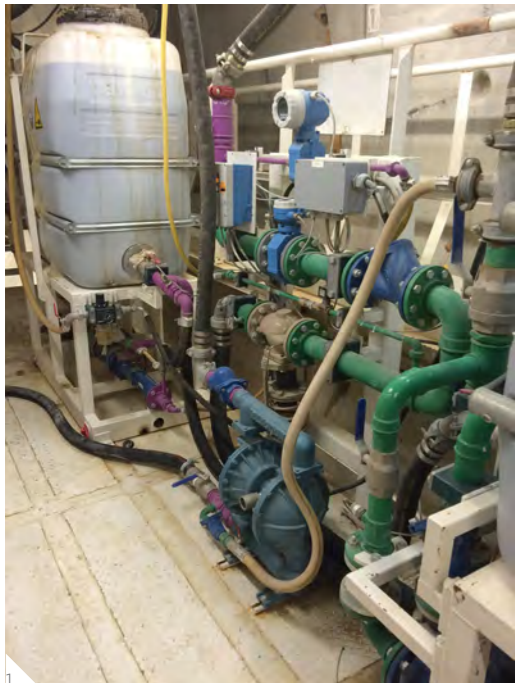
1-2 Sika TBM products during filling
