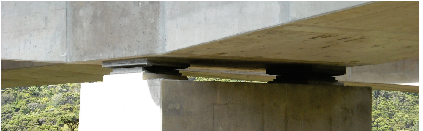
Sika Grout 212HP, a shrinkage compensated high strength cementitious grout, was then chosen to grout the bearing pads onto the piers.
