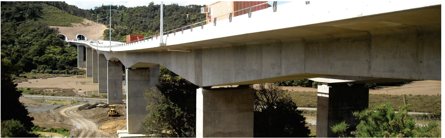
Sika ViscoCrete-20 HE and Sika ViscoCrete-2100 were used to achieve the necessary high early strength whilst allowing the concrete to flow through the congested steel to form the pre-cast panels.
