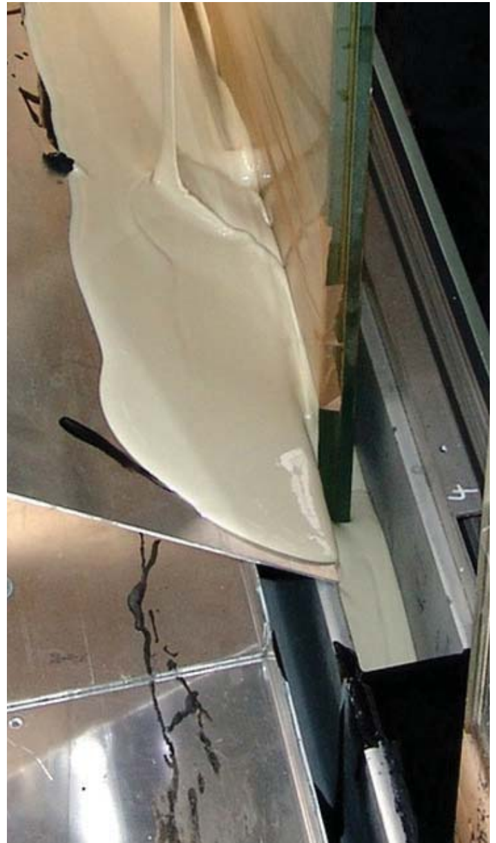
Picture 8: Easy injection of SikaGlaze GG-735 by using a sloped metal sheet
