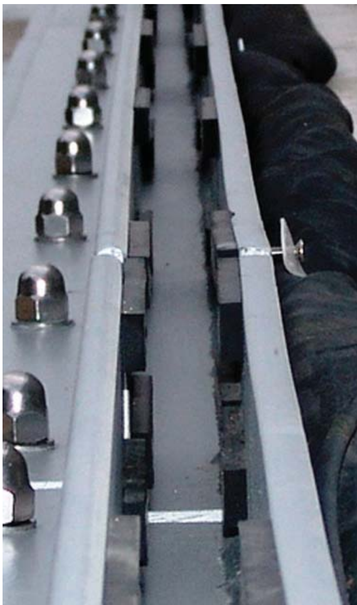
Picture 5: Glass fixing blocks in U-channel
