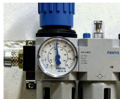
Fig. 13 Deoiler for compressed air
