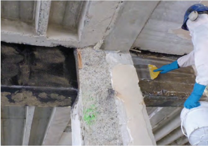
BBR Contech applied SikaWrap®-600 C woven carbon fibre fabric to provide additional shear strength and full confinement to the building's existing beam column joints.
