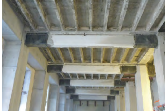
BBR Contech applied SikaWrap®-600 C woven carbon fibre fabric to provide additional shear strength and full confinement to the building's existing beam column joints.
