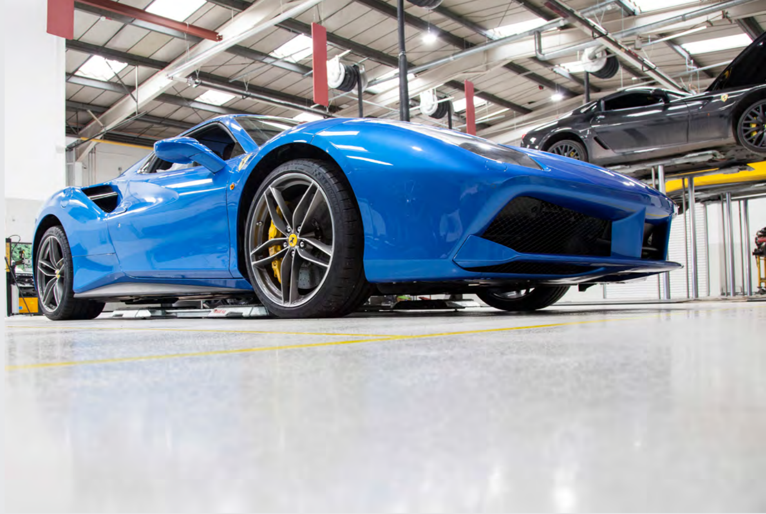
A light-grey finish with highslip resistance was applied.
