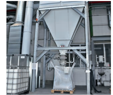
REUSE OF FILTER DUST IN PRODUCTION, SIKA GERMANY PLANT ROSENDAHL, GERMANY
