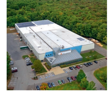
ENERGY SAVING PROGRAM AND SOLAR ENERGY SOURCING, SIKA CORPORATION PLANT CANTON, USA
