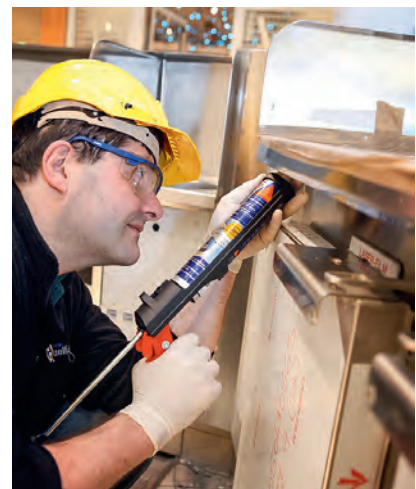
Fig. 9 Application of Sikaflex®-252
