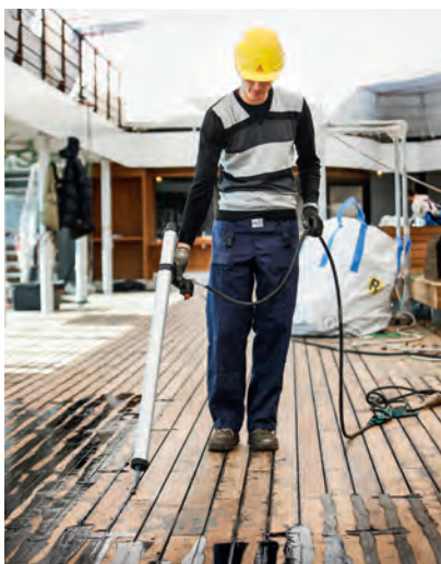
Fig. 17 Applying Sikaflex®-290 DC PRO
