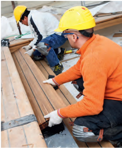
Fig. 13 Putting down the decking
