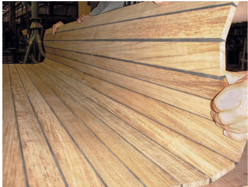
Fig. 23 Deep joint prefabricated teak decking and the strength and flexibility inherent in the adhesive
