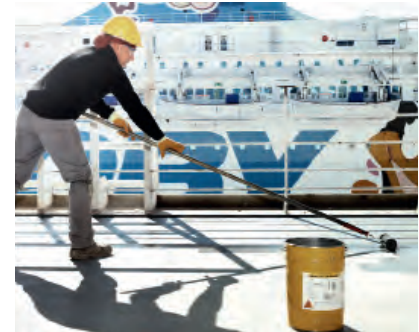
Fig. 3 Applying SikaCor® ZP Primer with a roller
