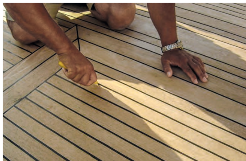
Fig. 34 Using a craft knife to cut along the part of the joint to be removed
