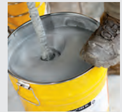
Fig. 5 Mixing SikaTransfloor®-352
