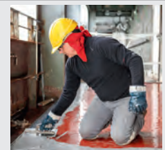
Fig. 8 Spreading the SikaTransfloor®-352 (SL/ST)
