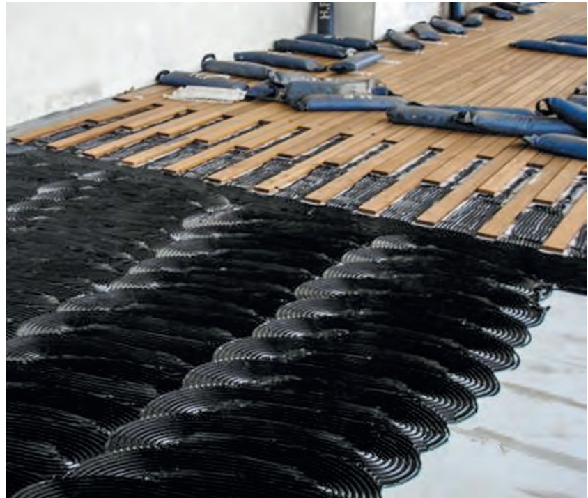
Fig. 14 A teak floor being laid, showing the bedding compound and the weights to hold it in place
