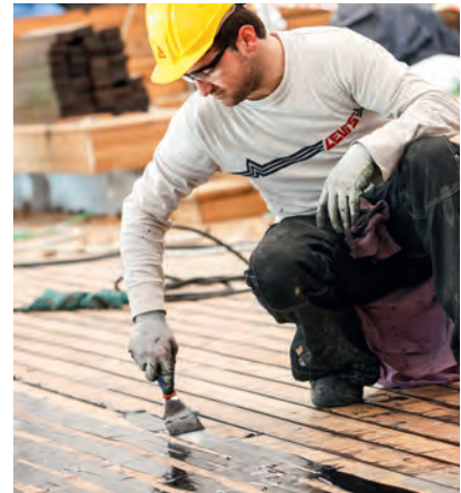
Fig. 19 Compressing Sikaflex®-290 DC PRO with a spatula
