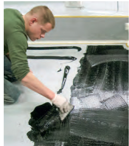
Fig. 55 Application of Sikaflex®-298
