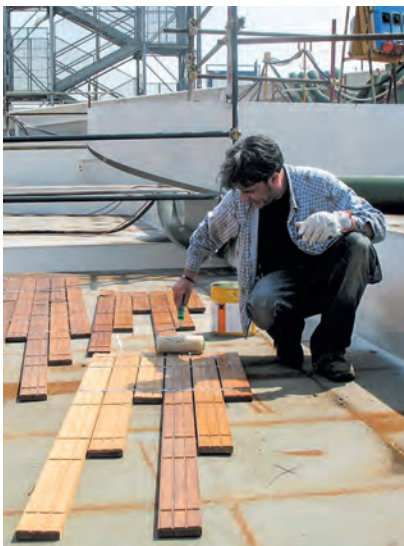
Fig. 9 Applying Sika® Primer-290 DC or Sika® MultiPrimer Marine to a teak deck with a roller (hidden side)
