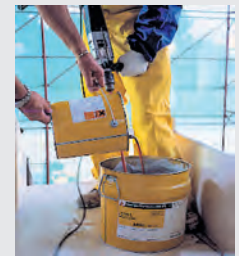
Fig. 6 Transferring the SikaTransfloor®-352 (SL/ST) to another container
